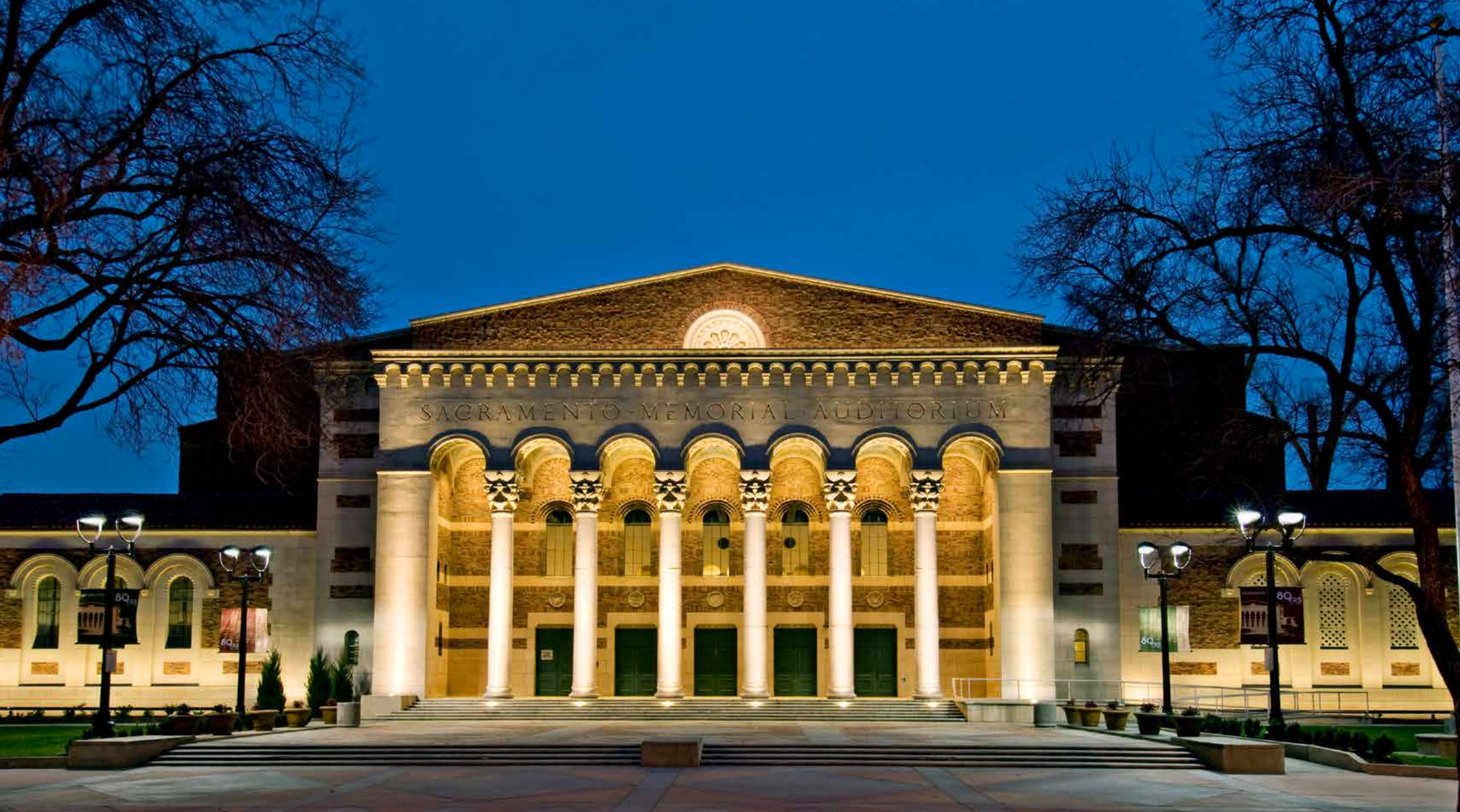
Sacramento Memorial Auditorium Products: 4750LCR Static White, 8100 Static White Floodlights, In-grades
