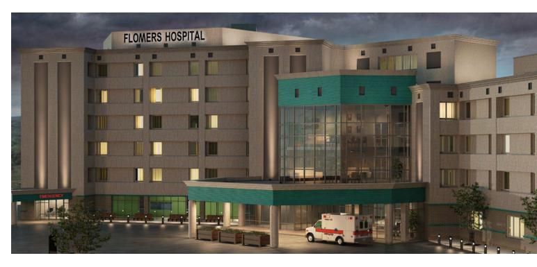
Floodlighting reinforces the architectural form by illuminating setback portions of the façade. In this example, the central vertical areas above each entrance and the top floor levels are illuminated while leaving the outer corner volumes unlit. The contrast between these surfaces emphasizes the solidity of the outer surface while accentuating the lighter interior volume that rises within and above.
