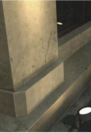
The 20 pilasters that run the length of this classically designed building are each up lit to emphasize their solid form. Lighting is positioned at the base of each pilaster in a recessed trough lined by ornate fencing. The SAF14 is easily tucked away to allow the architecture to speak for itself. With an IP68 rating, these luminaires will continue to perform even if those troughs become temporarily flooded.
